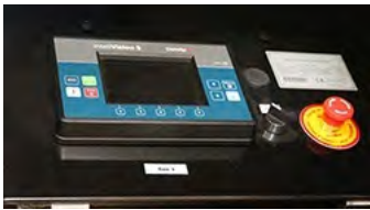
Comap IntelliGen Control panel
