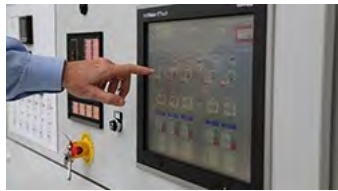
SCADA with IntelliTouch touchscreen
